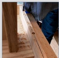
With the apron centered on the underside of the table top, pre drill and counter sink holes approximately every 8-12 inches apart, down the center of the  $2\frac{1}{2}$  inch apron sides. The apron will be attached to the underside of the table with 3 inch self tapping cabinet screws, digging into the table top about  $\frac{3}{4}$  of an inch.
